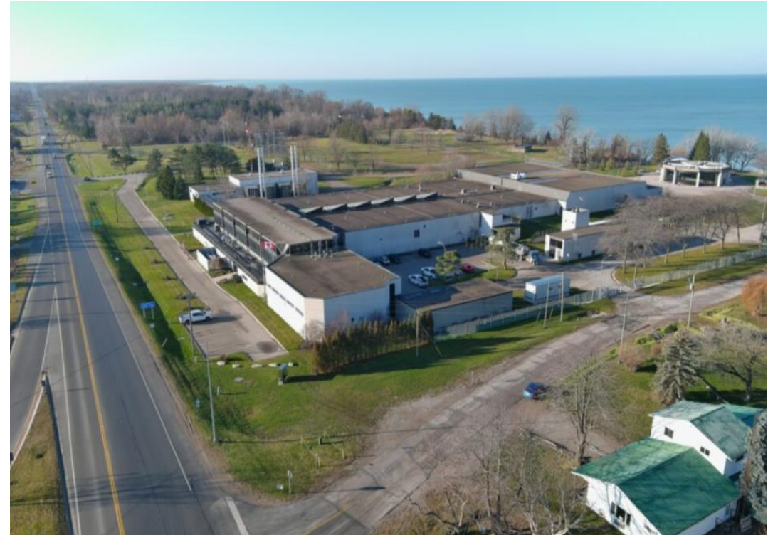
Lake Huron Primary Water Supply System facility
